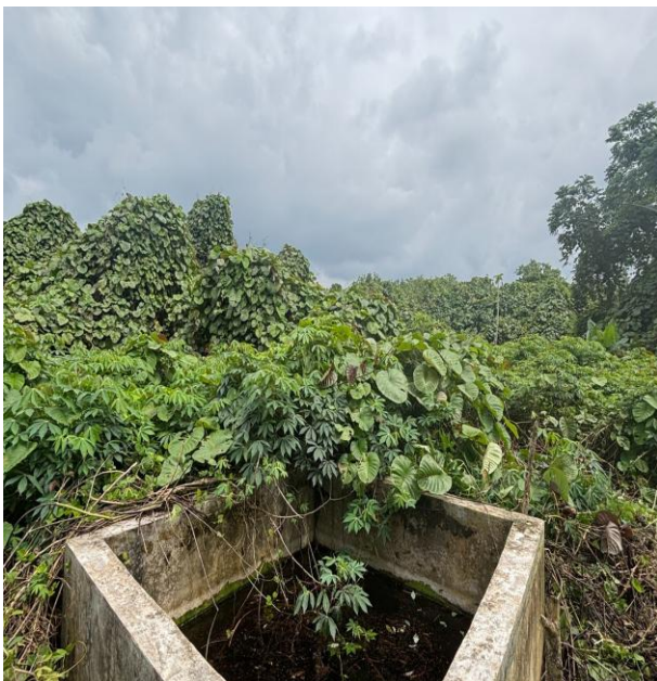
Existing water-related concrete structure observed
