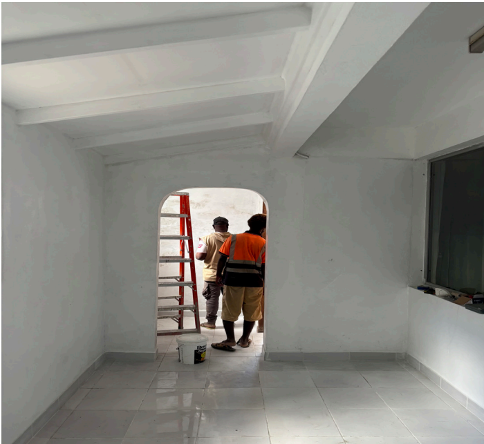
Local Workers Supporting VFIPA's Head Office Expansion
