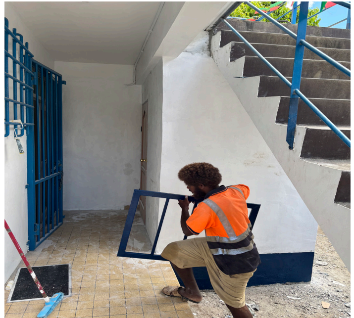
Local Workers Building VFIPA's Expanded Workspace
