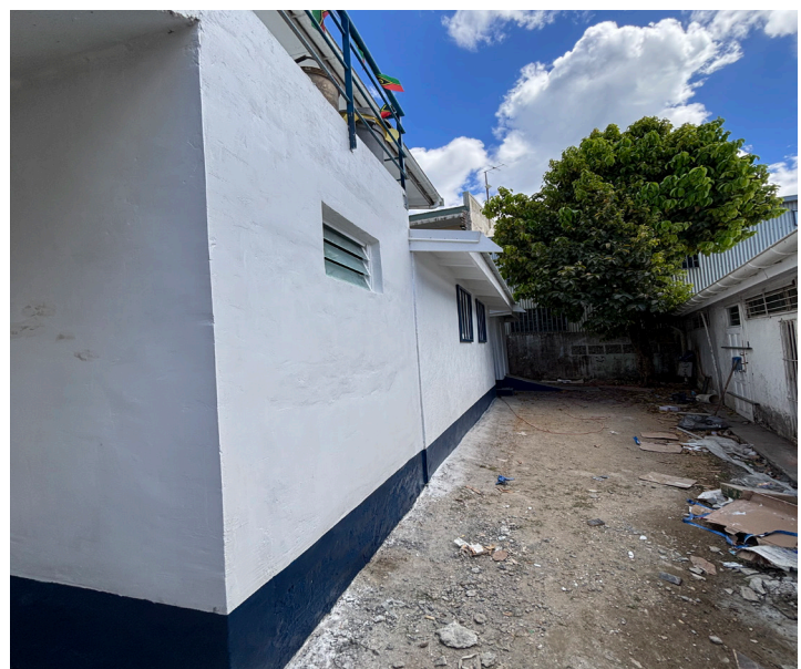
Construction Progress at the Back of VFIPA's Head Office
